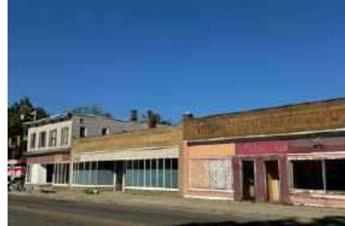
A vacant commercial building.
