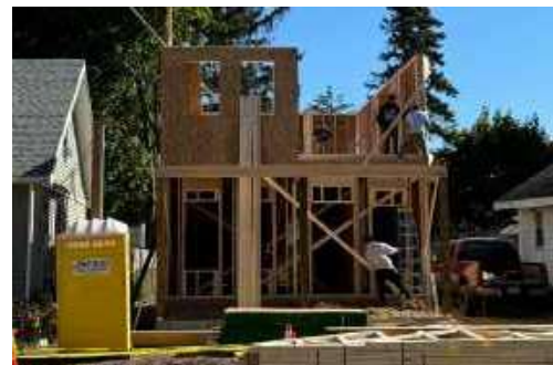
A home under renovation.
