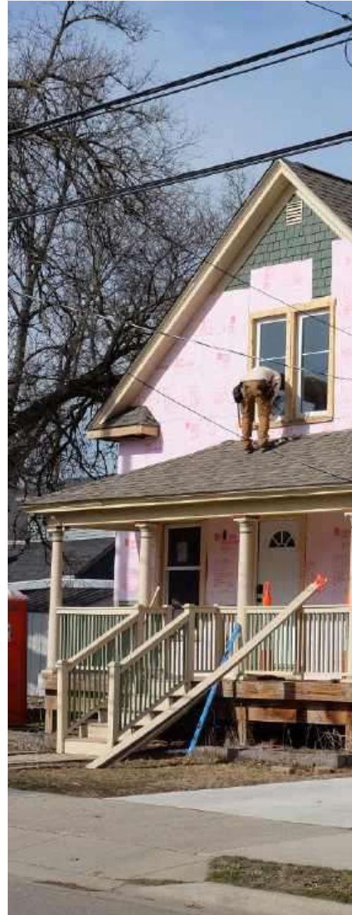
A home currently being renovated in Southtown.
