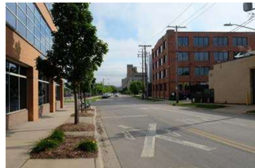
Office and research buildings along the riverfront.
