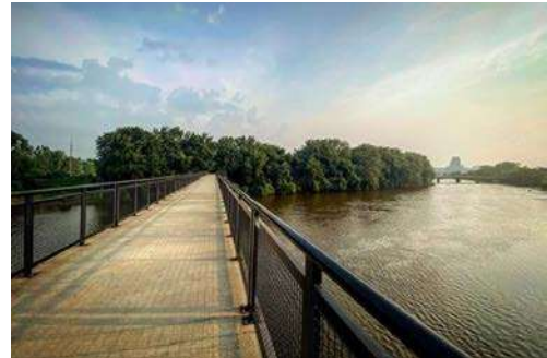
Oxford Trail bridge crossing the Grand River.
