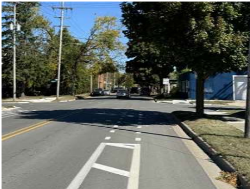
Existing bicycle facilities on Butterworth Street.
