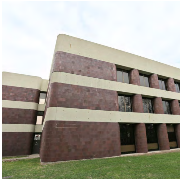
Obsolete building at corner of College and Fountain
