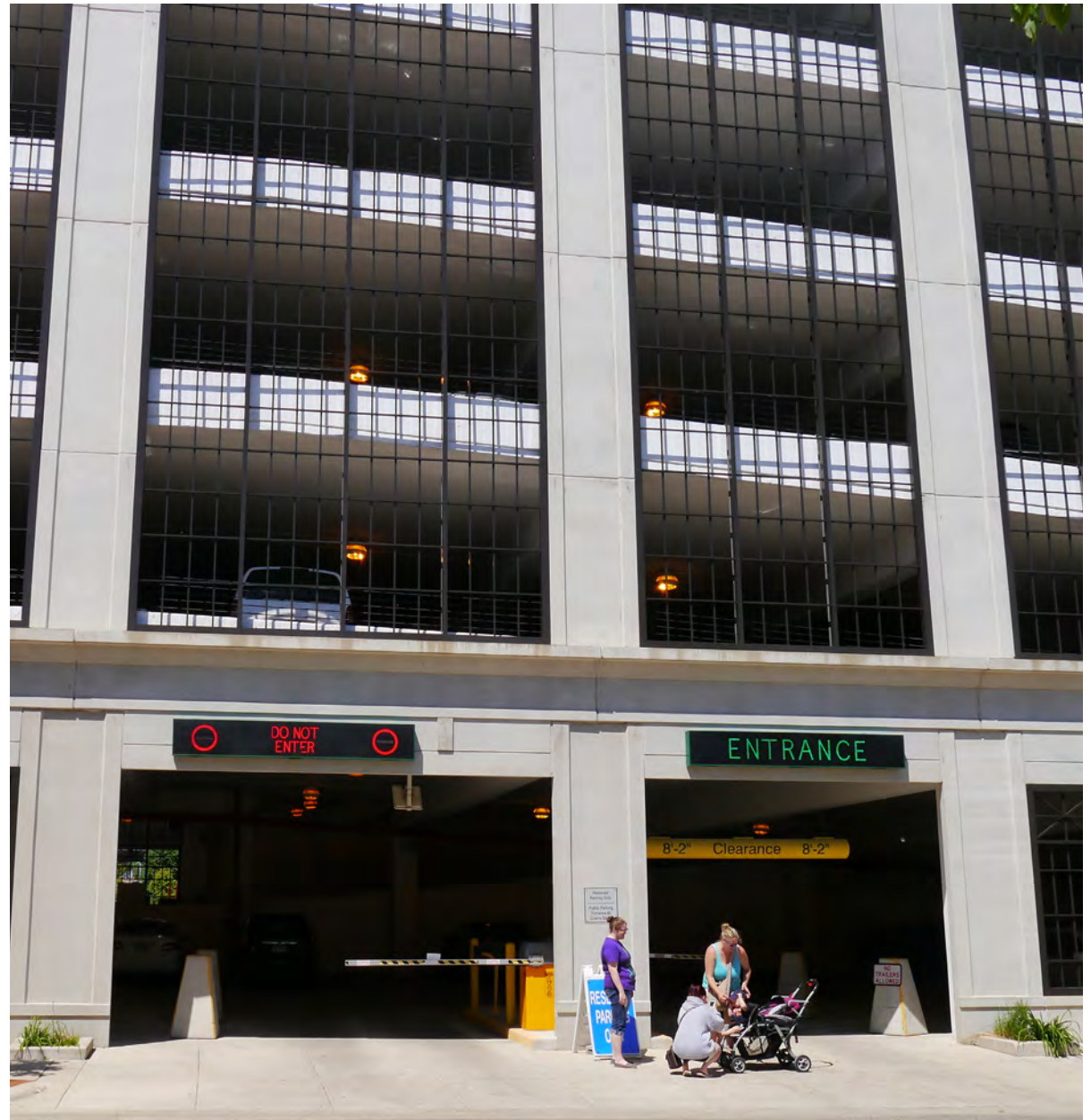
Existing parking facility facade
