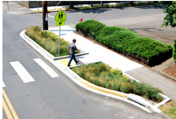
Planted curb bump-out with integrated storm water management
