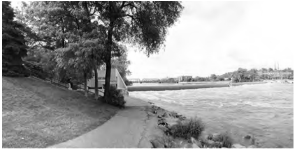
Existing river trail at the Fish Ladder
